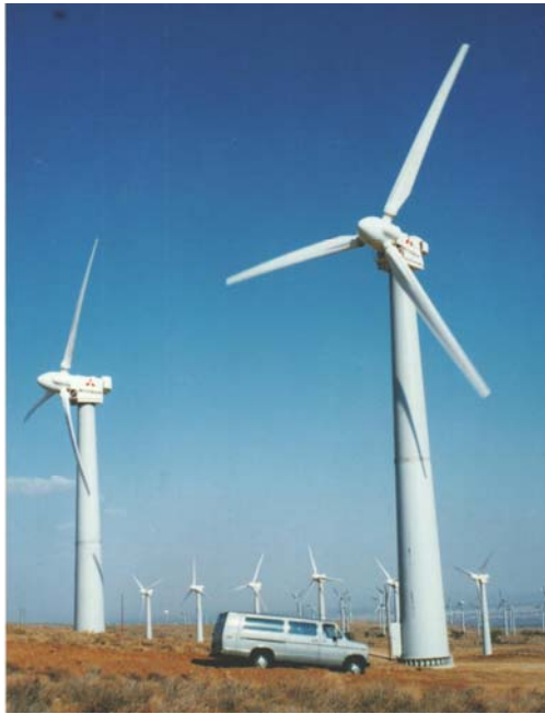
Fig.7.13 250kW Wind turbines and GFRP blades (Length: 12m)
