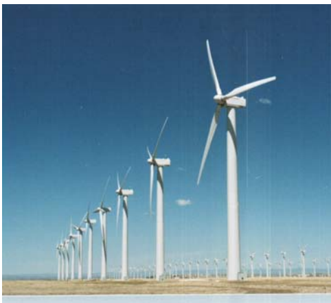
Fig.7.14 600kW Wind turbines and GFRP blades (Length: 18m)
