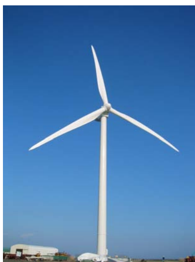
Fig.7.16 2400kW Wind turbine (Blade Length: 45m)
