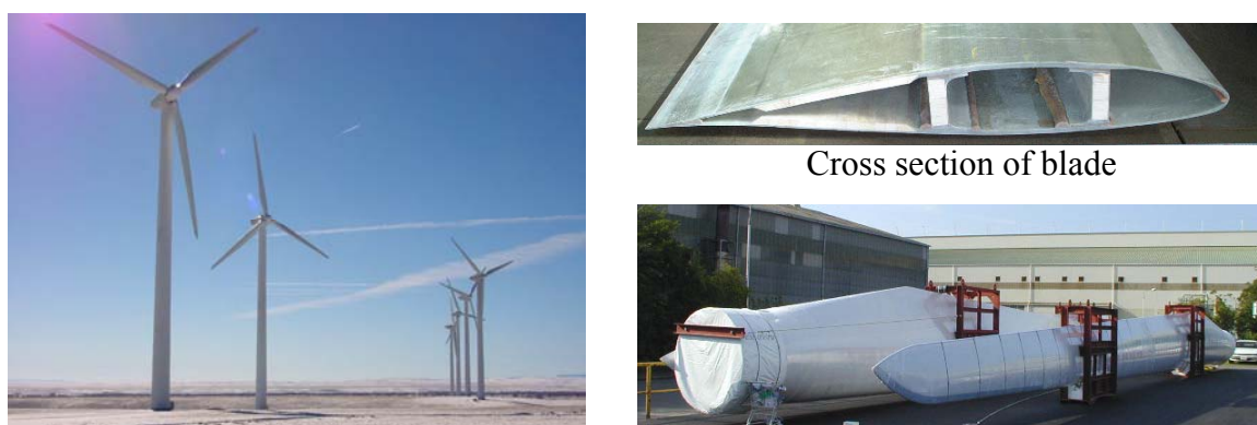
Fig.7.15 1000kW Wind turbines and GFRP blades (Length: 27m)
