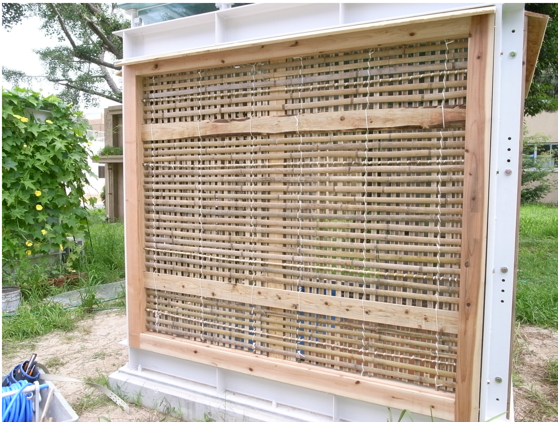
Fig.4-1 Woven Take-Komai Made of Bamboo on Shikkui Cube
