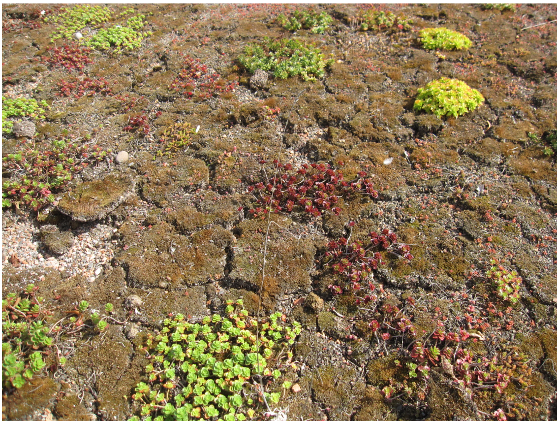
Fig.3-4 Unplanted Mosses at the Brown/Biodiverse Roof at Royal Holloway, University of London
