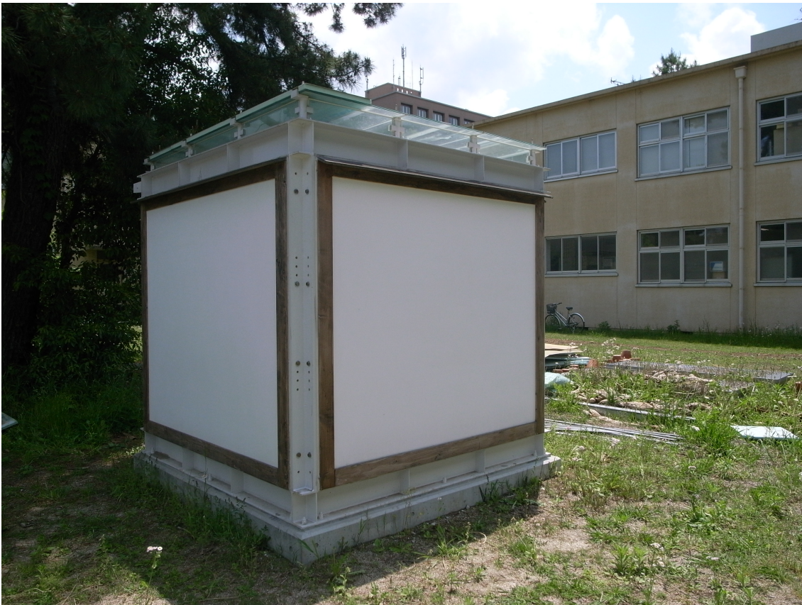
Fig.4-2 Completed Shikkui Cube
