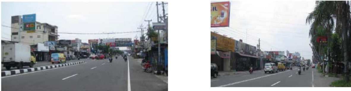
Figure 4: Parangtritis(Yo) and Solo(Yo) Road Section Condition in Yogyakarta Municipality
