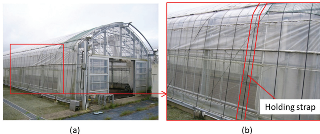
Figure 2. (a) Greenhouse with fully opening roof and (b) straps used to hold the plastic film and roll-up system in place.
