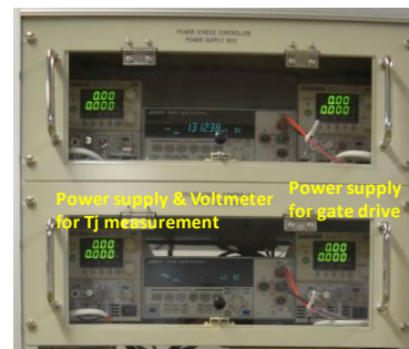
Fig. 4. Power supply box.
