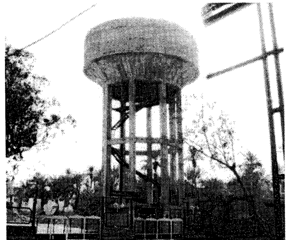
Photo 11 Water tank in the severely damaged area
