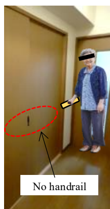
(a) Sliding door without handrail
