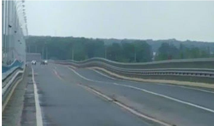
Figure 1.1.1 Vortex-induced vibration in the Volgograd Bridge 1)
