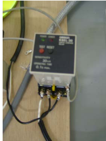
Figure 11 ZCR Relay
